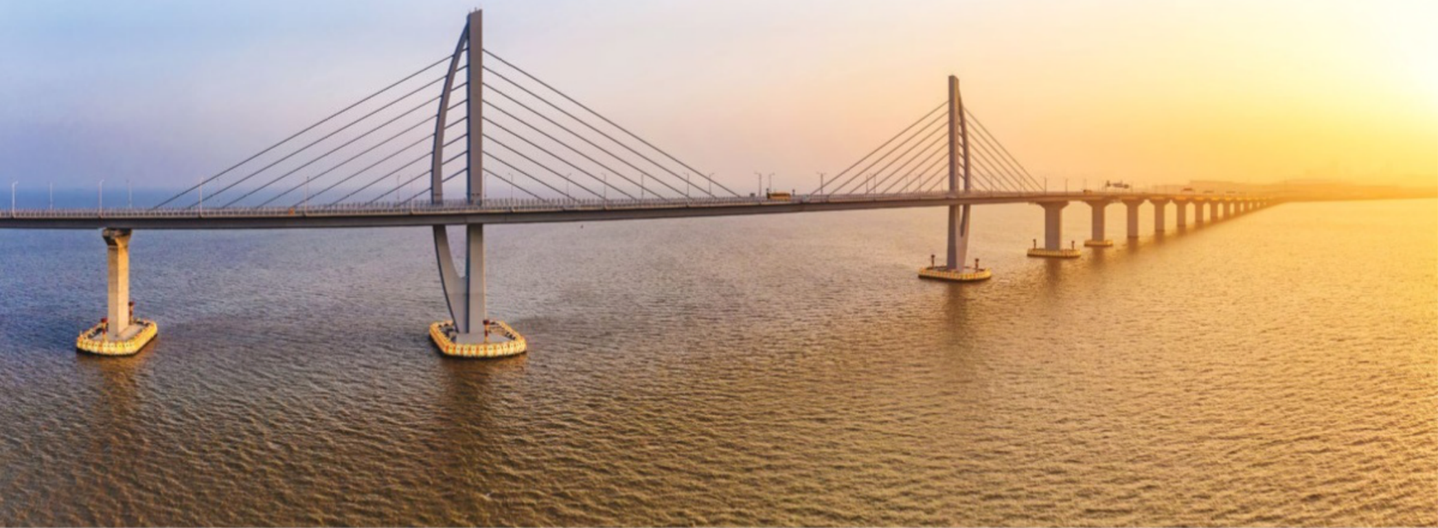
Hong Kong-Zhuhai-Macao Bridge
